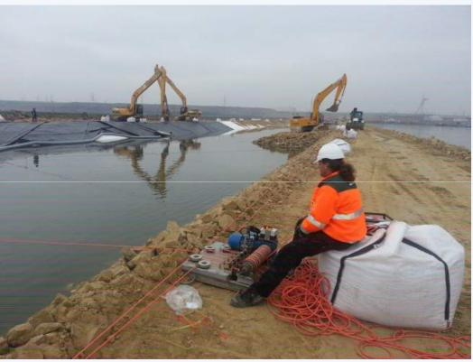
Geomembranes, winches and cables for positioning before submerging under water
